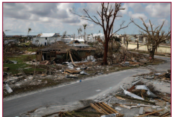
Destruction caused by Hurricane Dorian on Abaco and Grand Bahama islands.
