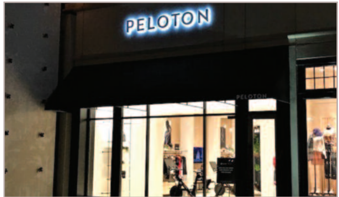
Peloton , Houston, TX Superintendent: Rich Carlton Project Manager: Colton Remakel
