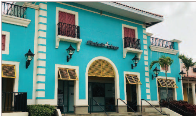
Finish Line , Barceloneta, PR (Hurricane Rebuild) Superintendent: Charles Kirtley Project Manager: Jay Saterbak
