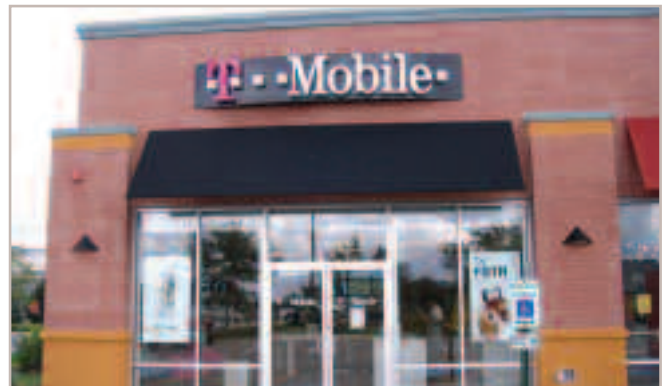
T-Mobile , St. Charles, IL Superintendent: Terry Blank Project Manager: Jason Ash
